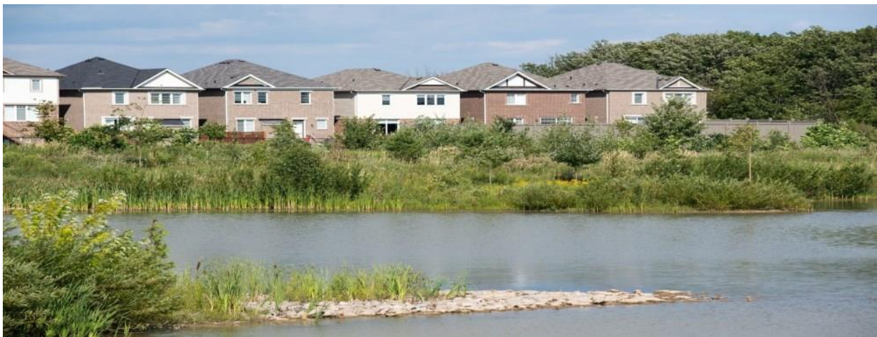
Figure 3 Open stormwater Pond in Milton
