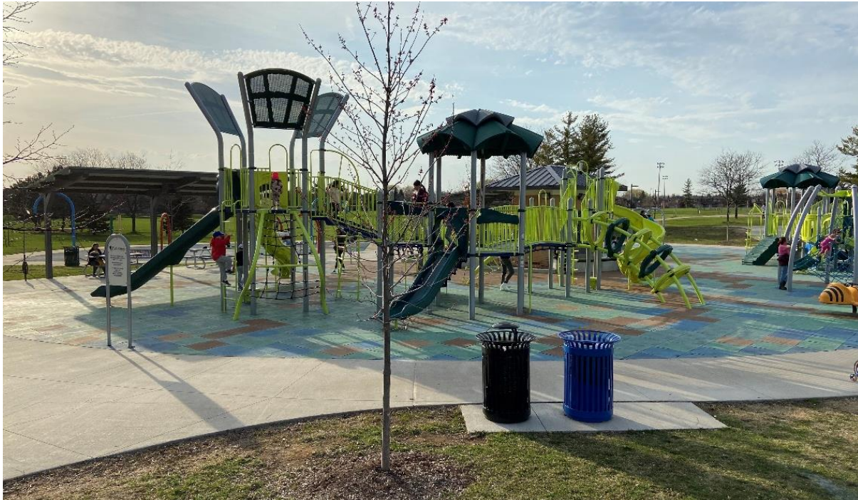
Figure 7 Playgrounds can be built on top of DUSFs
