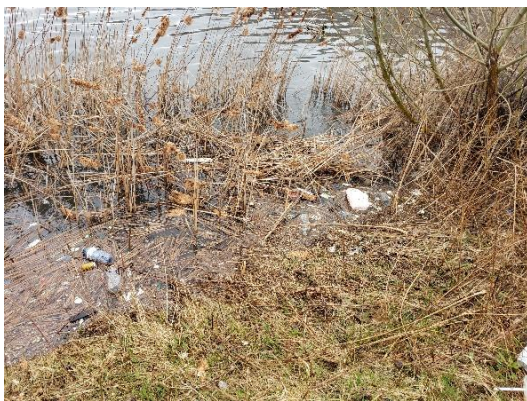
Figure 5 Example of debris in the stormwater pond
