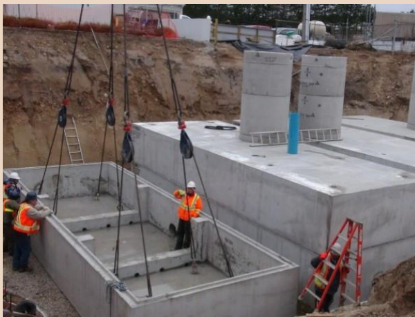
Figure 1 Underground Storage Facility Installation
